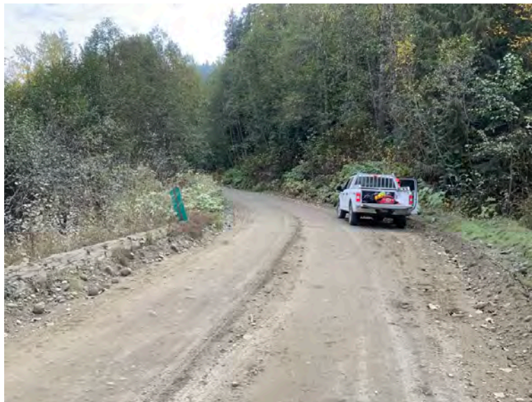
Right Bank Abutment when facing downstream
