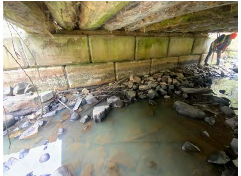
Right Bank Abutment when facing downstream
