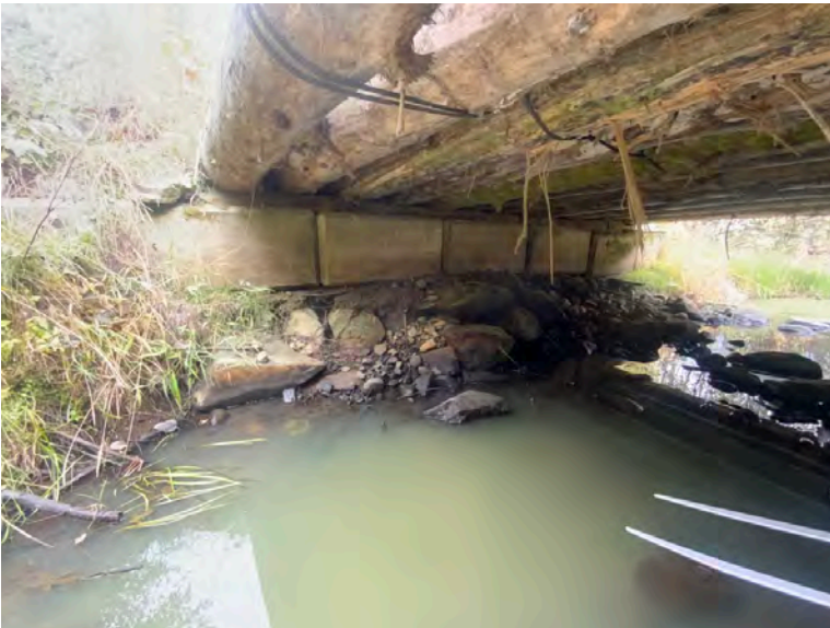
Right Bank Abutment when facing downstream
